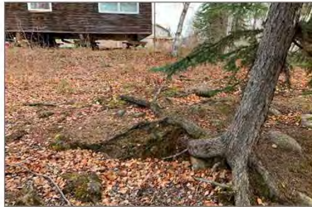
Photo 43: Photo R2-5A (top) from EBA (2006)/ 2021 Photo 43 (bottom). House 1S, facing east. Tension crack mostly unchanged located approximately 9 m from the corner of the house, increased leaning of the foreground tree, some erosion around base of tree.
