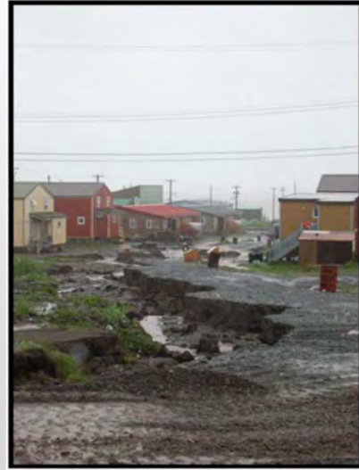
Erosion after major rainfall event (Kugluktuk, July 2007)
